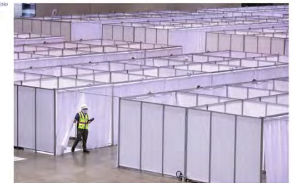
Construction at the COVID-19 field hospital at McCormick Place in Chicago on April 16. The city opened back space for a 3,000-bed temporary hospital as the nation's largest convention center as infection numbers decreased.
